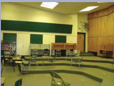
Stepped concrete Band Room floor
