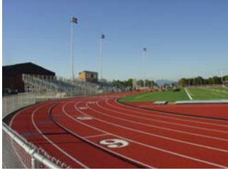
Phase I Athletic Fields, Parking Drainage and Site Utilities (2003)
