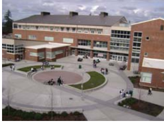
Phase II New Main Classroom Building and Campus Commons (2005)
