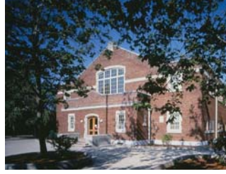
Phase II Original Gym Building converted to Fine Arts (2005)
